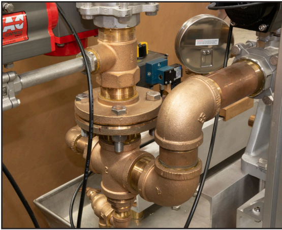
Figure 6 - Outlet Valve Assembly
