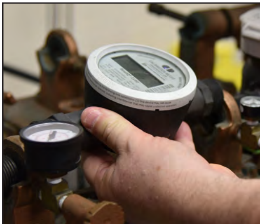
Figure 2 - Install water meter
