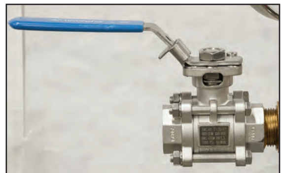
Figure 7 - Bench Inlet Ball Valve (shown in the open position)
