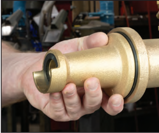
Figure 1 - Install meter adapters and gaskets
