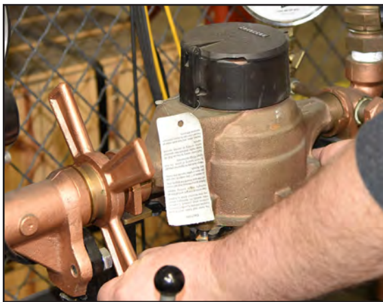
Figure 2 - Install water meter
