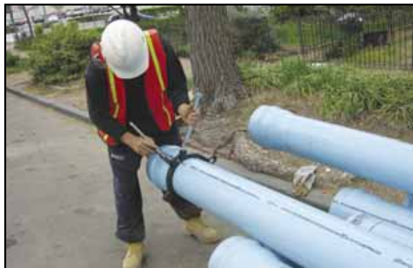
Uni-Flange 1390s can be pre-assembled on PVC pipe, allowing fast installation.
