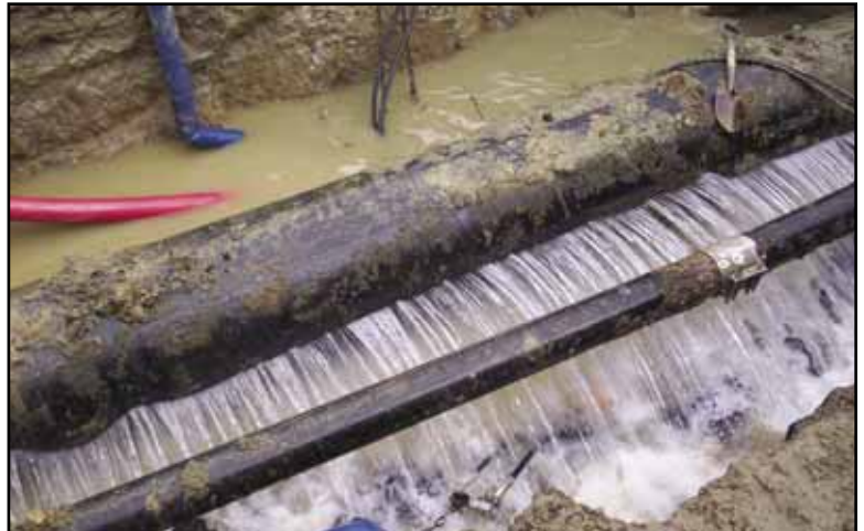
A very rare full-length break of a 24" water main.
