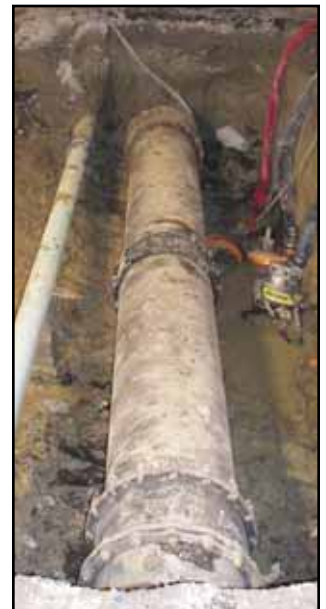
The fix is complete with couplings and new pipe.
