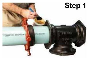
Before installation, be sure to clean the sealing surface areas of the pipe and the mechanical joint socket.
