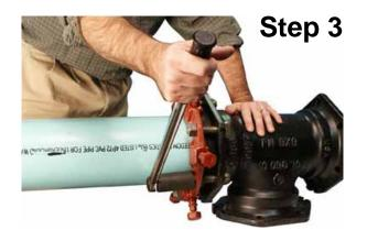
**Step 3**. Tighten the tee bolts in an alternating manner to ANSI/AWWA C111 specifications. Use of a torque wrench is recommended.
