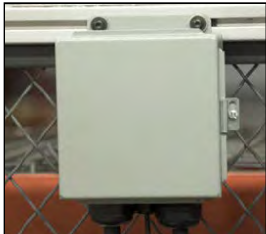
Figure 7 - Return Pump Relay Box
