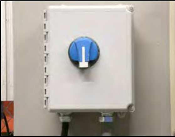
Figure 8 - System Safety Disconnect
