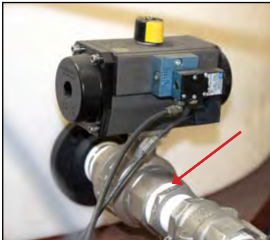
Figure 5 - Measuring Tank Outlet Valve
