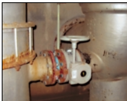
AFTER - a new backwash valve installed using a Uni-Flange® Series 900 Flange Adapter
