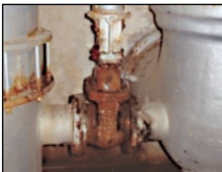
BEFORE - an old backwash valve requiring change-out
