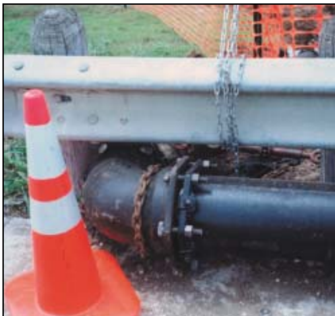
An eight inch Uni-Flange® 1400 locks a ductile iron water main to an elbow. The emergency water main was chained in critical areas to prevent shift and movement.
