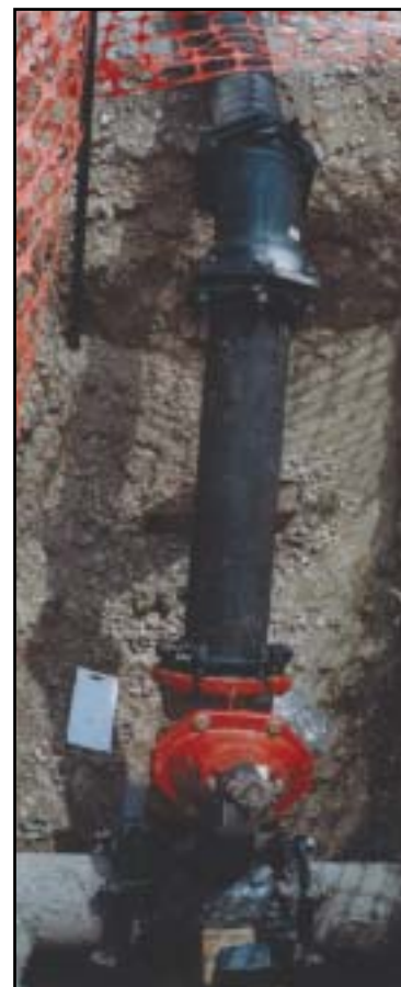
The Uni-Flange® 1400 restrains components of the temporary above-ground water main.
