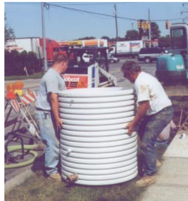
Contractors lower an inch and a half meter setting into place in Delaware, Ohio
