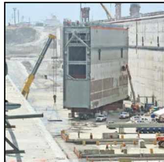
A massive canal gate is moved into place.
