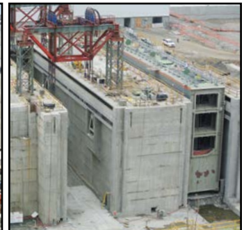
A massive canal gate is moved into place.
