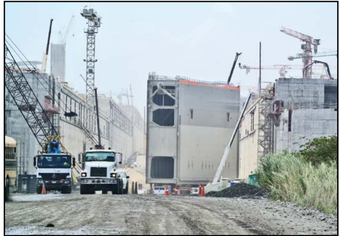
A massive canal gate is moved into place.
