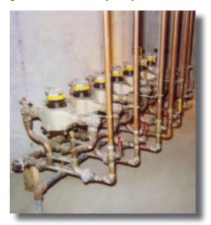
This sub-metering manifold setting installed in New Boston, Michigan greatly reduced the space normally required for an apartment complex.
