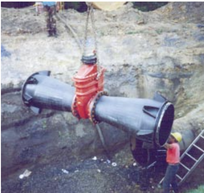
A 24" resilient seat gate valve attached to Ford fabricated concentric reducers is lowered into the trench.
