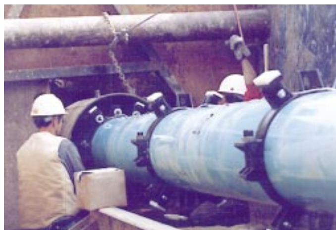
A Uni-Flange UFRCS1390 installed at the joint is shown as it enters the casing. Also shown installed are two UFRCS1300s. These fittings are installed to provide support of the pipe between the joints.
