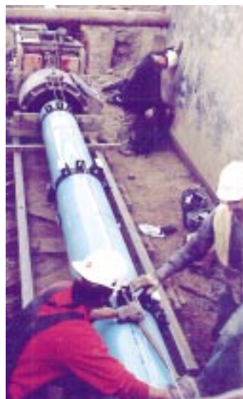
The crew makes final adjustments to the pipe before installation into the casing.
